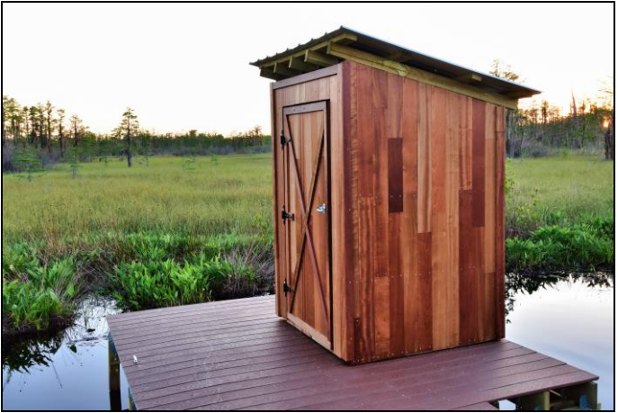
Every campsite and day-use shelter has a vault/pit toilet. Pictured: Cedar Hammock.
