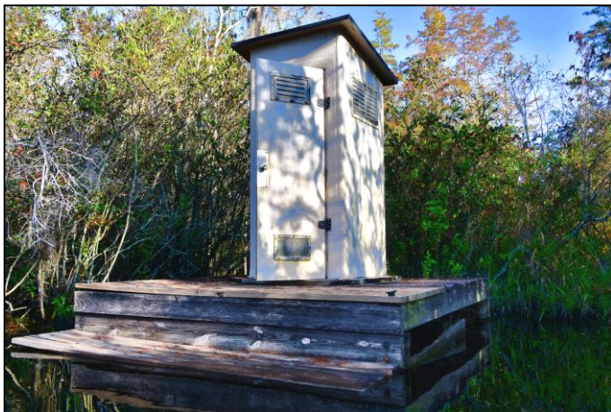
Pit toilet on small platform on the Suwannee Canal / Orange Trail.
