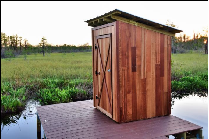
Every campsite and day-use shelter has a vault/pit toilet. Pictured: Cedar Hammock.
